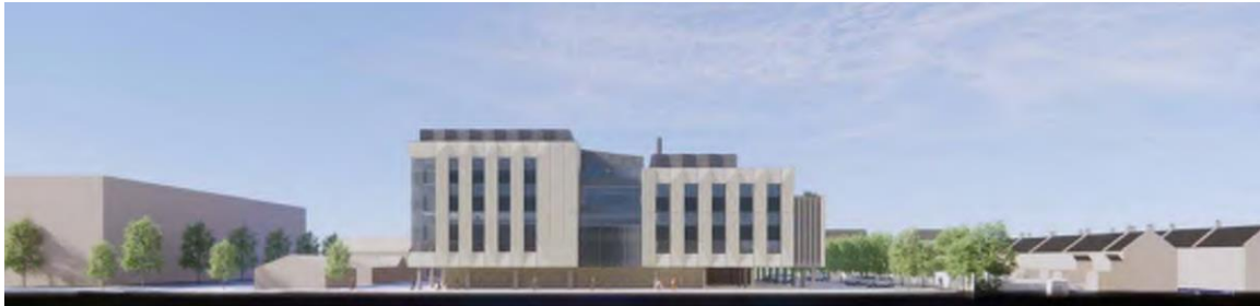
Figure 5 – image of rear (south) elevation
